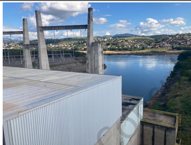
Photo 2: View from Aimorés HPP powerhouse (330 MW) to Rio Doce and Baixo Guandu town
