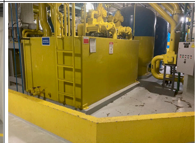
Photo 48: Oil containment barrier for unit 2
