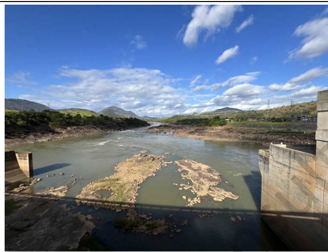
Photo 62: View from central dam downstream, with powerhouse release from right and spillway on left
