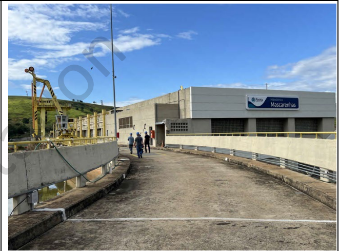
Photo 27: Road across top of concrete dam
