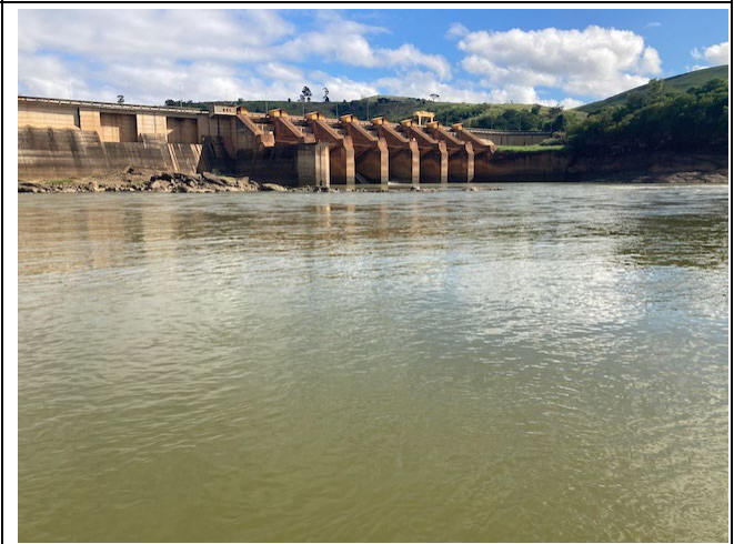
Photo 30: Spillway from downstream
