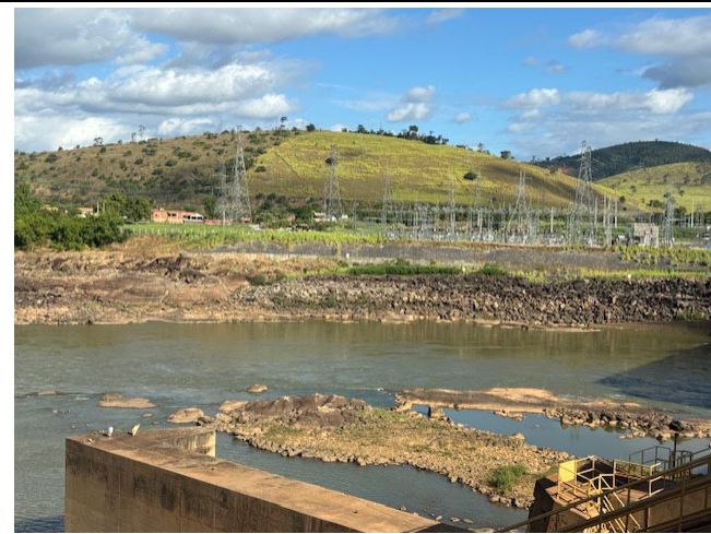
Photo 67: Substation with Vila Mascarenhas behind
