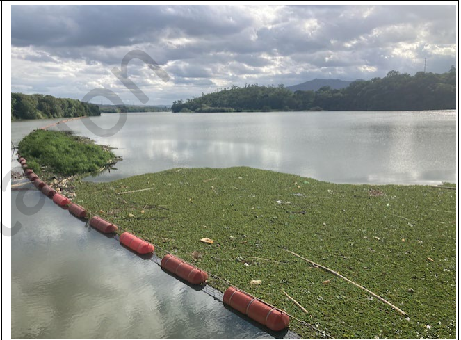
Photo 9: Log boom above intakes with minor accumulation of macrophytes
