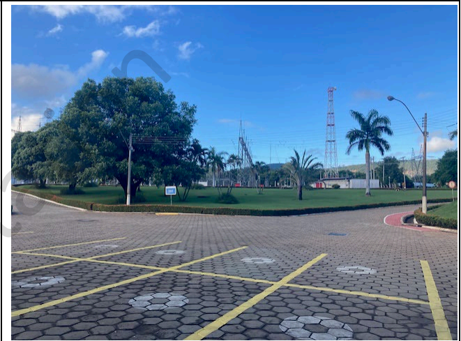
Photo 21: Landscaping and signage between powerhouse and substation
