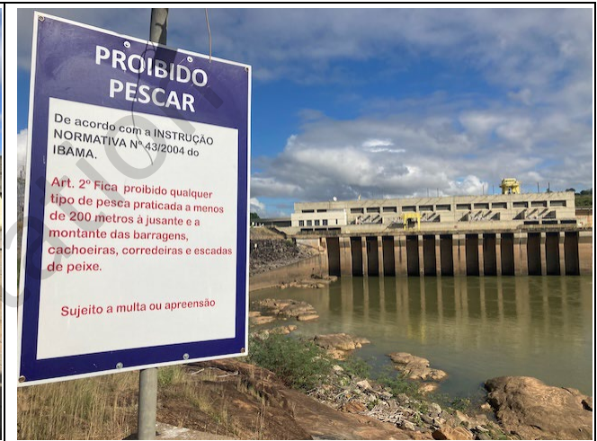
Photo 63: Fishery exclusion zone close to power plant
