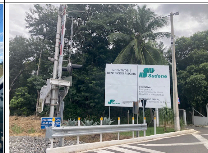
Photo 18: Railroad crossing signal and sign for tax benefits next to entrance to power plant
