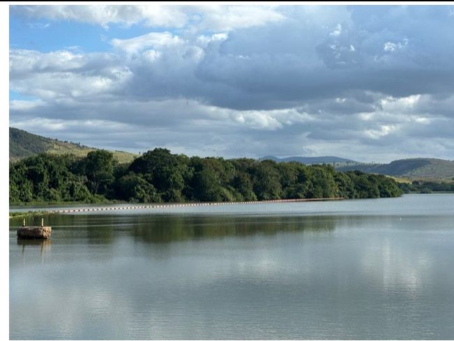
Photo 7: Right bank of the reservoir
