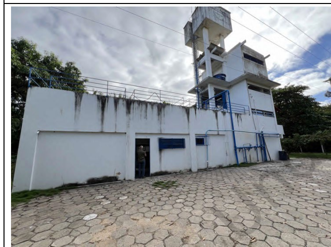
Photo 16: Water treatment facility originally built for project and now operated by municipality
